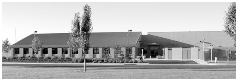
BFS Central Valley Regional Laboratory in Ripon, CA.
